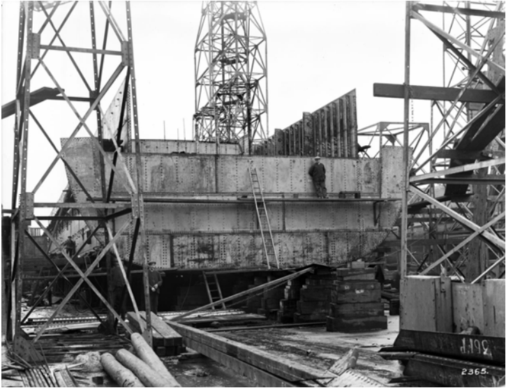
A Section of the SS Oranjestad at the beginning of construction Note the flat bottom.
