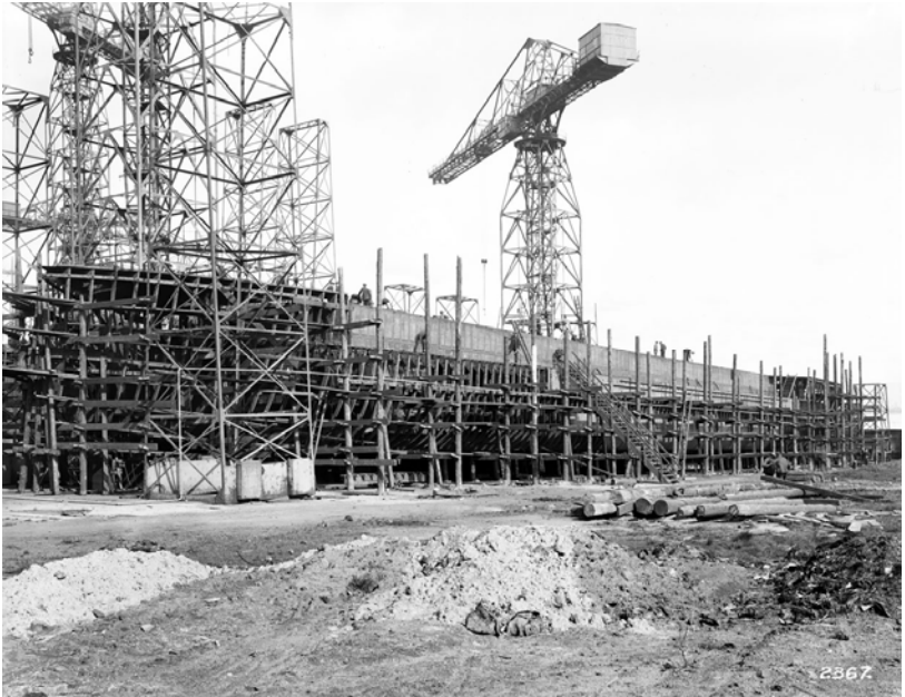
Here you can see the ship's ribs as the steel skin is applied.
