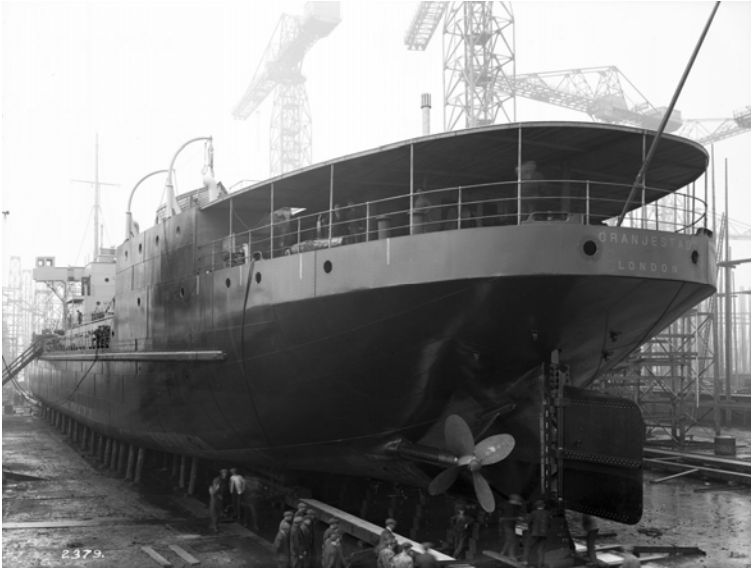
The aft of the ship on the dry dock ways, with a good view of the propeller that was later salvaged. Note how the propeller is tucked up above the flat bottom to protect it when the ship hit crossing the sand bar at the entrance to Lake Maracaibo.
