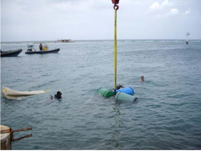
Just before the lift, drums and air bag are still attached
