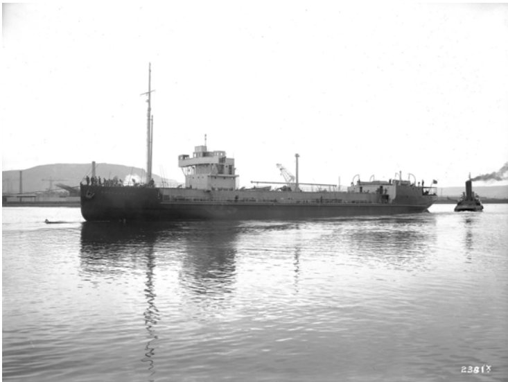
An unfinished SS Oranjestad is towed up river for additional work.
